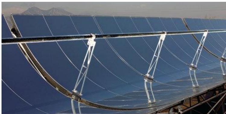
Figure 3C.3 Parabolic trough
