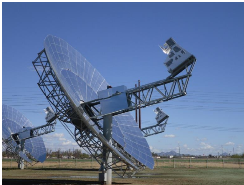
Figure 3C.5 Dish/engine system
