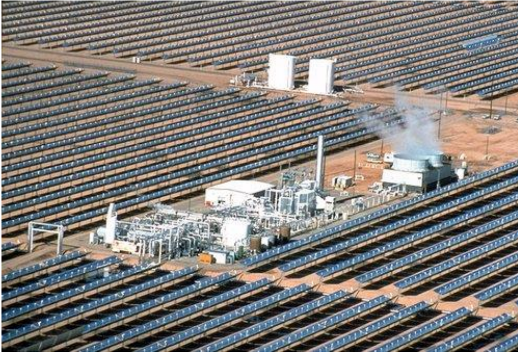
Figure 3C.4 Linear collector system
