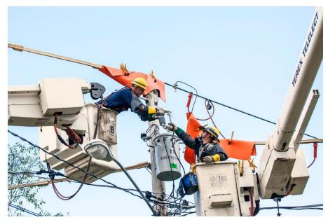
devices in order to remove electrical hazards from disturbed or fallen lines or to facilitate repairs
